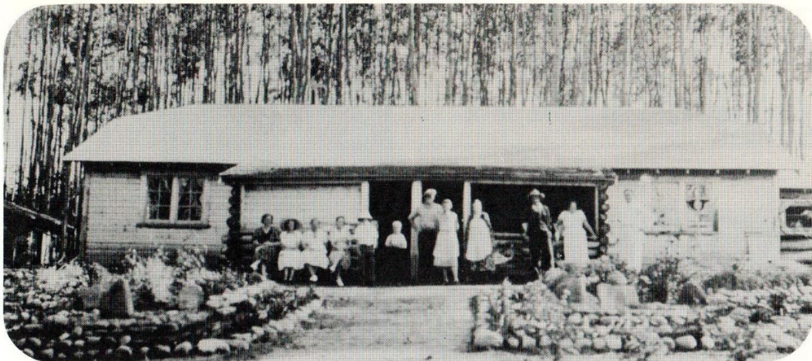
The original dining hall viewed from the north side. Note the extensive rock garden in the foreground.
