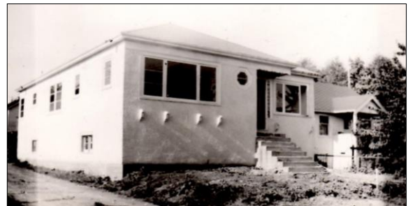
The house on Laurel Street
