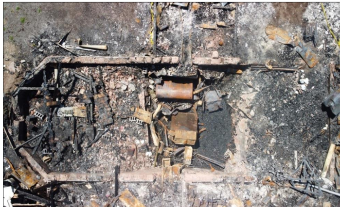
View after the fire, taken by a drone
