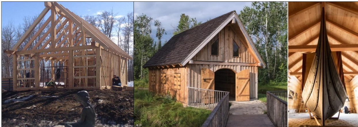
Building of the Naust from frame to completion and the Freydis Joanna in her new home
