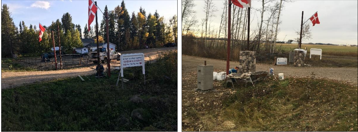
Removal of trees and construction of the new fence and gate
