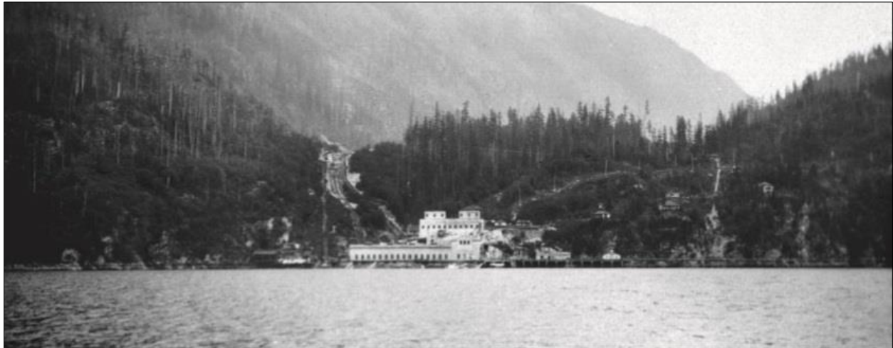
The power generating station on Buntzen Lake
