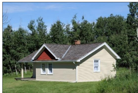
Right photo: The Nielsen CPR House after its restoration
