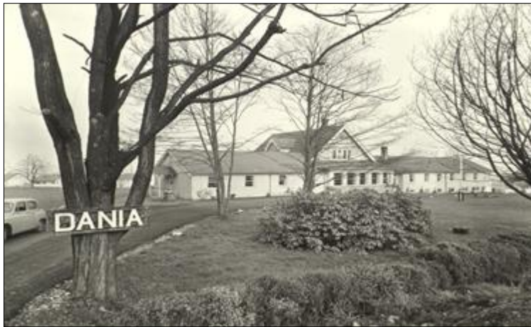
Original building with two new wings added on.
