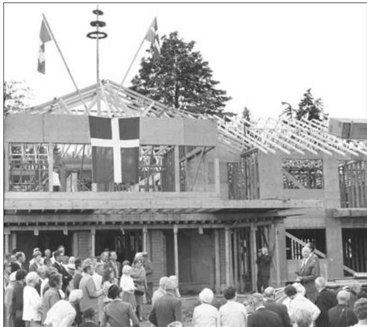
Carl Mortensen Manor (CMM) under construction
